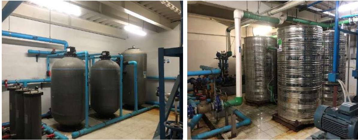
Figure 2-10 Raw Water Treatment System
